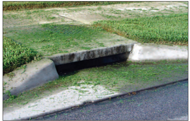
Figure 15. Always remove clippings from impervious surfaces. These nutrients are going straight to a water body.
