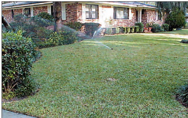
Figure 8. Poor design; system does not match irrigation requirements. The area needs to be rezoned with landscape and turf separated.
