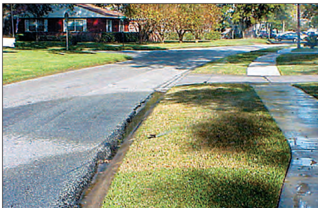
Figure 7. Poor design; sprinkler does not match area.
