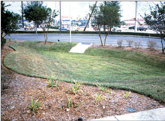
Figure 2. Grassy stormwater retention areas can add to a lawn and protect our environment.
